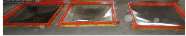
Fig.2 Moulds of Shallow Funicular Shells
