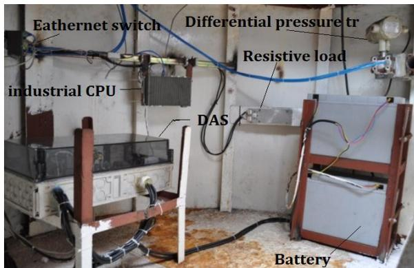
Fig5.2 Electrical & Instrument system inside BBDB
