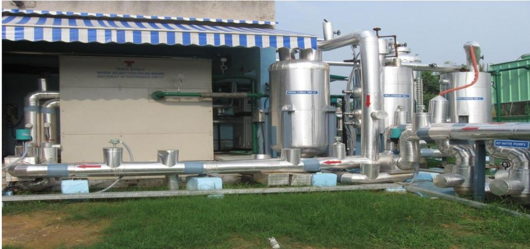
**Fig. 1. Pictorial view solar vapour absorption cooling system at NSI, Gurgon, Haryana, India**
