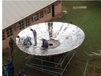
**Fig. 10:** Ensuring a perfect parabolic surface
