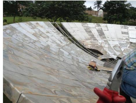
**Fig. 11:** The parabolic surface being covered by aluminium sheet
