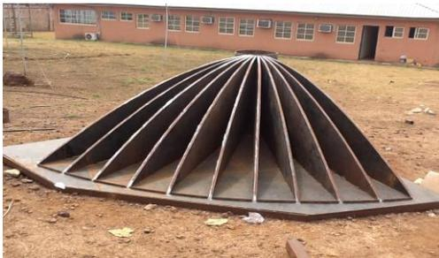
**Fig.7:** The finished mould for the ribs with a height of 1m.
