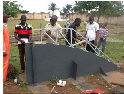
**Fig. 5: Forming a rib on its Mould**
