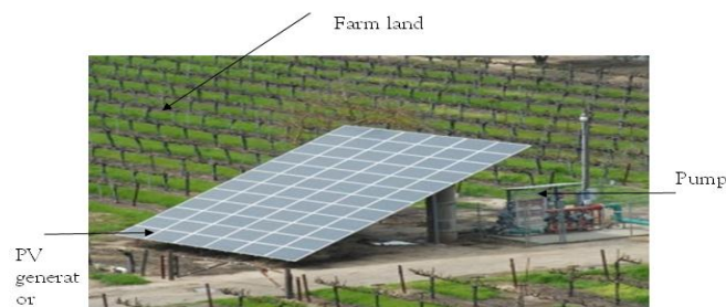
Figure 1: PV pumping System configuration
