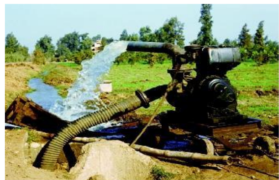
Figure 2: Pumping of water
