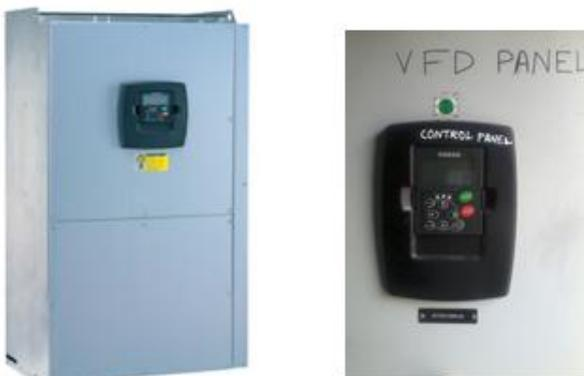
**Fig.6 photographs of VFD used in stacker/reclaimer LT drives, rating of VFD is 55kw,115A,415V.[13]**
