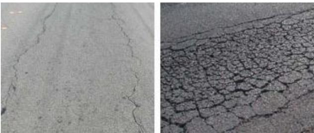
**Figure 3 Fatigue cracking on asphalt pavements [10]**
