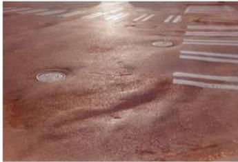
**Figure 2 Shoving of asphalt pavement [10]**
