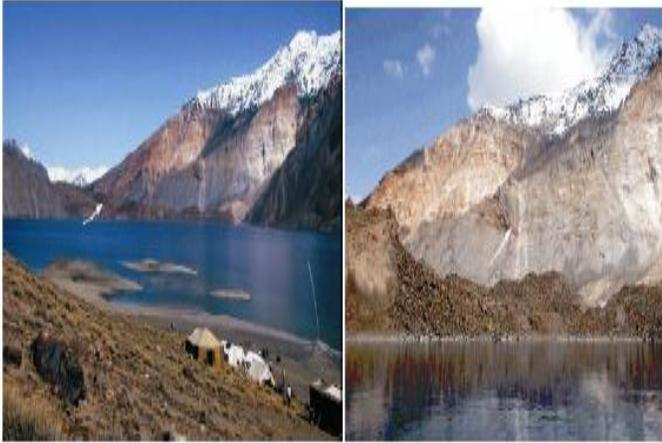
Fig. 2: Usoi landslide dam and Lake Sarez formed by 1911 earthquake in Tajikistan (dam height ca. 650 m; freeboard ca. 50 m; dam volume ca. 2 billion m<sup>3</sup>, world's largest dam) (Courtesy J. Hanisch)
