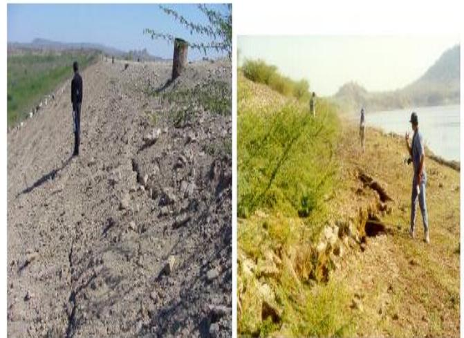
Fig. 1: Cracks in downstream (left) and upstream faces (right) of two damaged embankment dams, 2001 Bhuj earthquake (Courtesy Prof. S. K. Jain)
