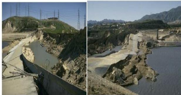
Fig. 3: Lower Van Norman Dam, a 38 m high hydraulic fill dam, experienced widespread liquefaction and major slope failures during the 1971 San Fernando earthquake, California (Courtesy Steinbrugge Collection, Earthquake Engineering Research Center, University of California, Berkeley)
