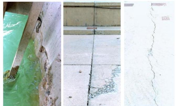
Fig. 4: Crack at upstream face of Sefid Rud buttress dam (left) and cracks in dam crest caused by the 1990 Manjil earthquake, Iran (Photos M. Wieland)
