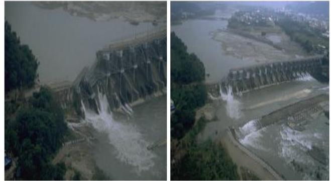
Fig. 5: Local damage of Shih-Kang weir due to large fault movement near right abutment, 1999 Chi-Chi earthquake, Taiwan (Courtesy C. K. Yeh)
