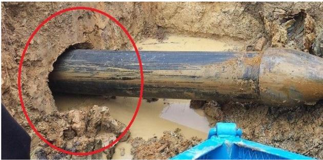
**Figure 4. Overcut created by folded CMP**
